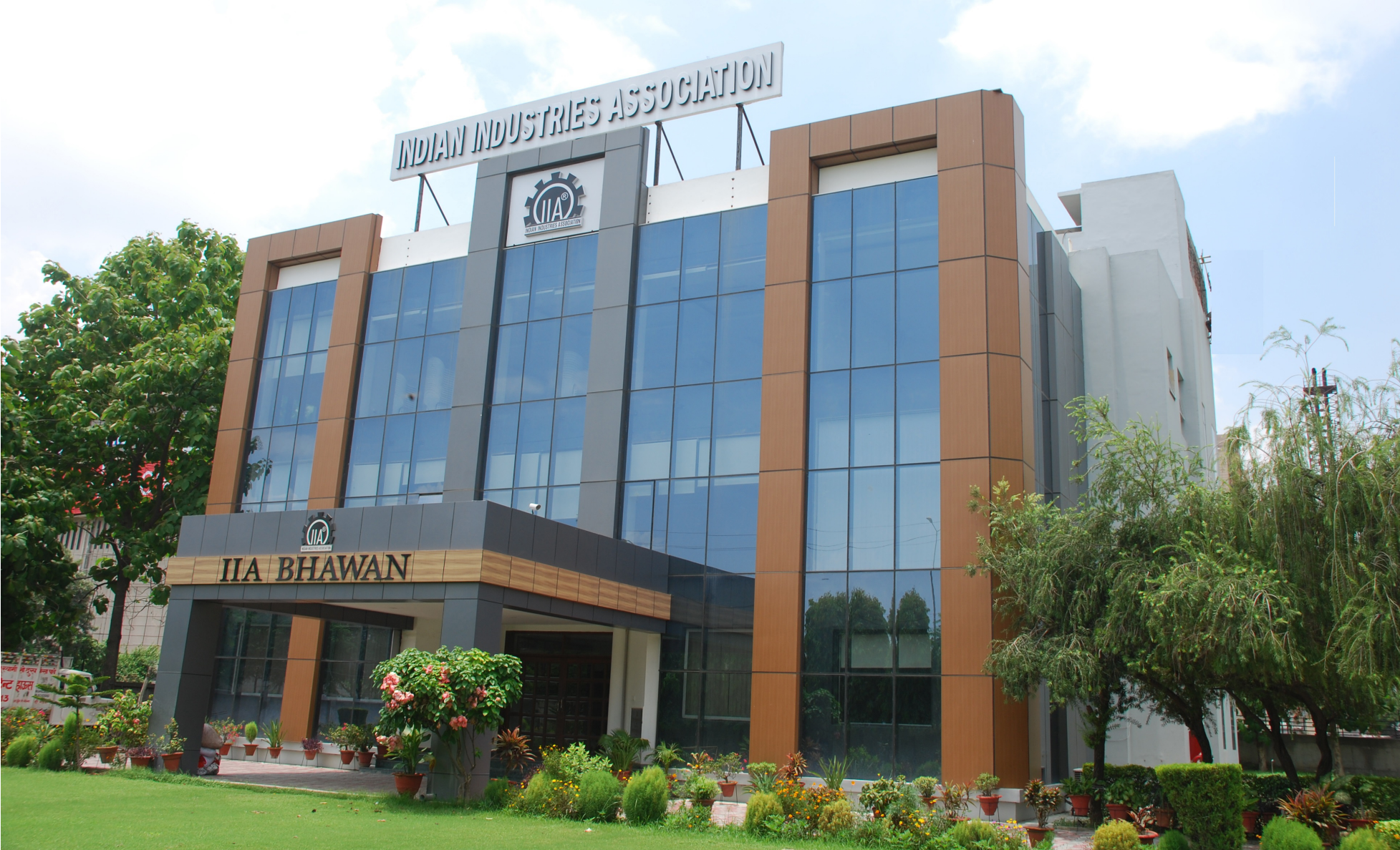
IIA Existing Building
