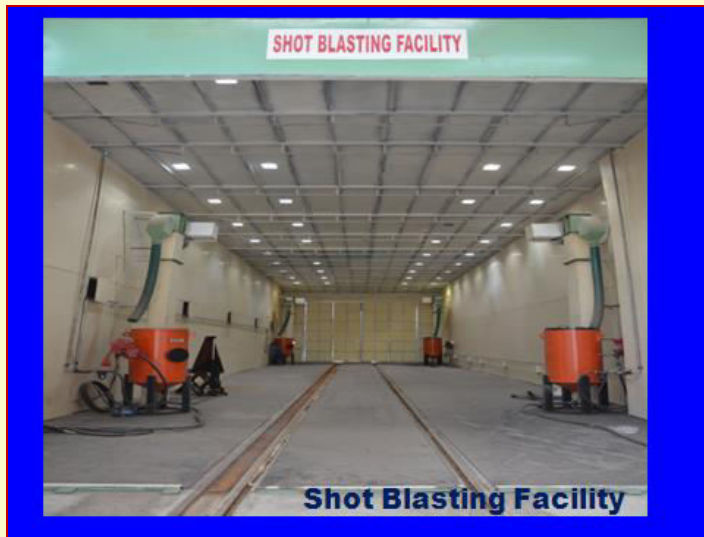
SHOT BLASTING FACILITY
